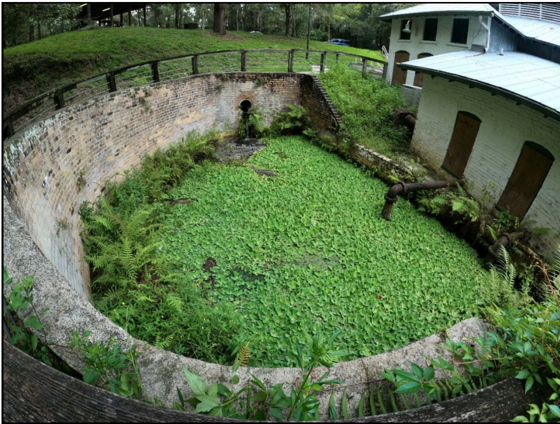
Photo 8. Boulware Spring head pool; the spring vent is to the left at the base of the wall opposite the intake pipe.
