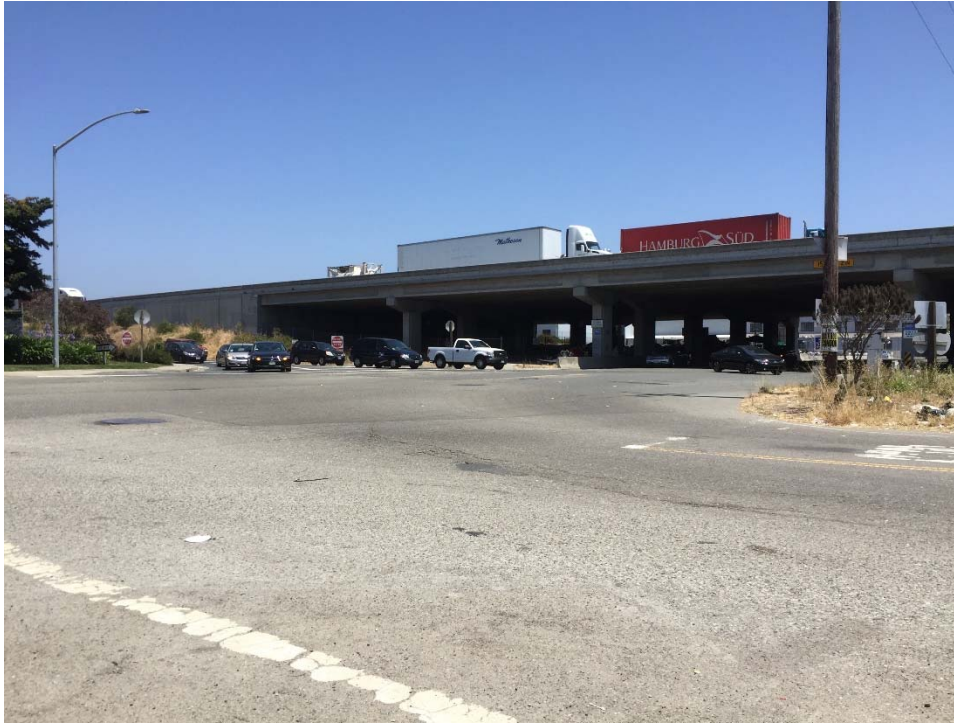
Photo 9. Looking East toward I-80/Gilman Street Interchange from San Francisco Bay Trail
