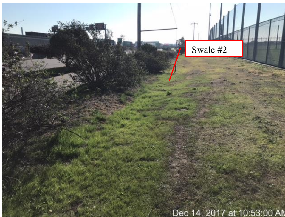
Photo 6. Swale Conditions on December 14, 2017, Looking South.
