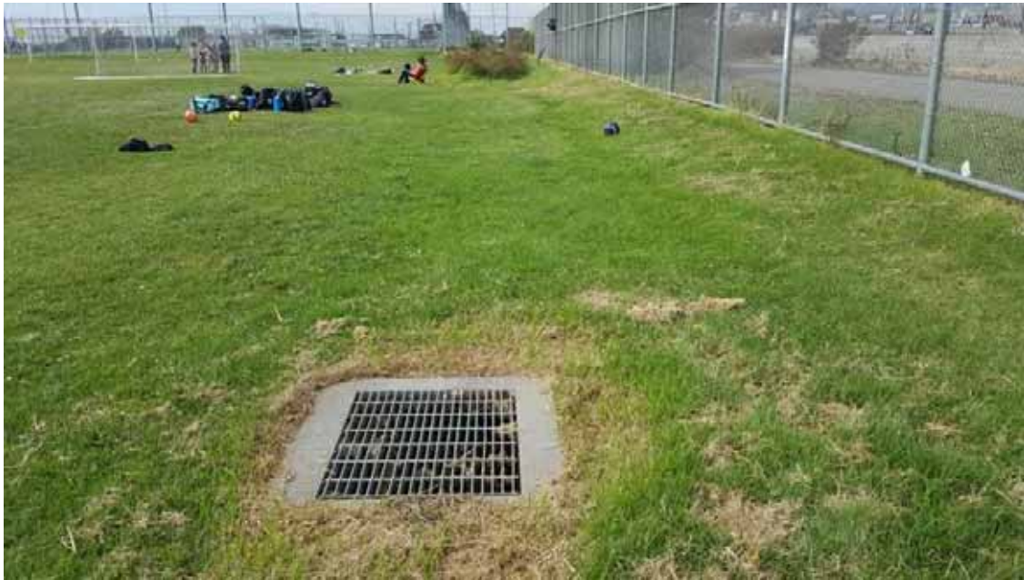
Photo 5. Drainage Grate South of Depression 1, facing north
