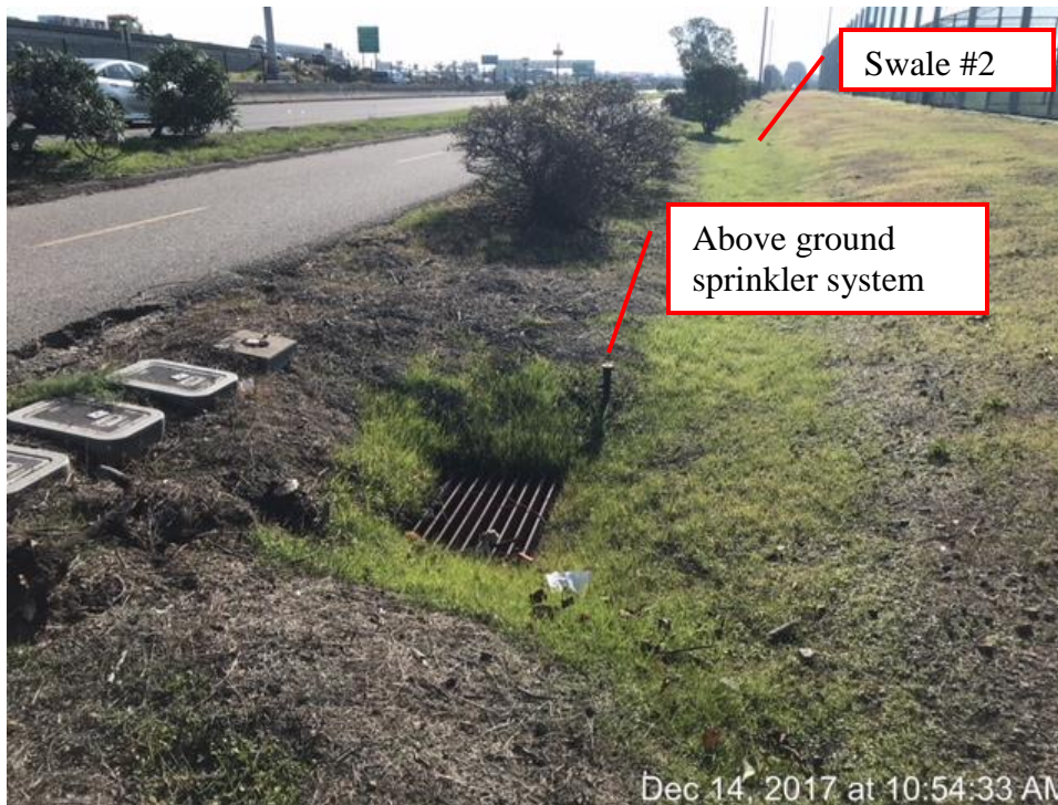
Photo 5. Drainage Inlet along Swale #2, Looking South.
