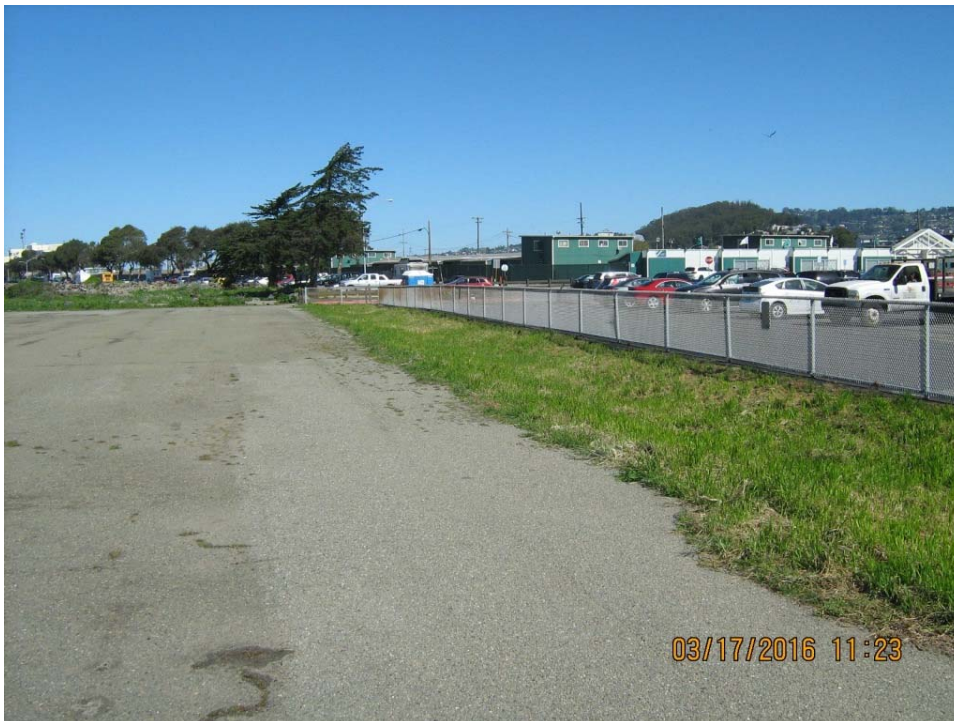
Photo 4. Looking North toward 60-inch Culvert Outfall, Stables at Golden Gate Fields, and Parking Lot at Tom Bates Sports Complex
