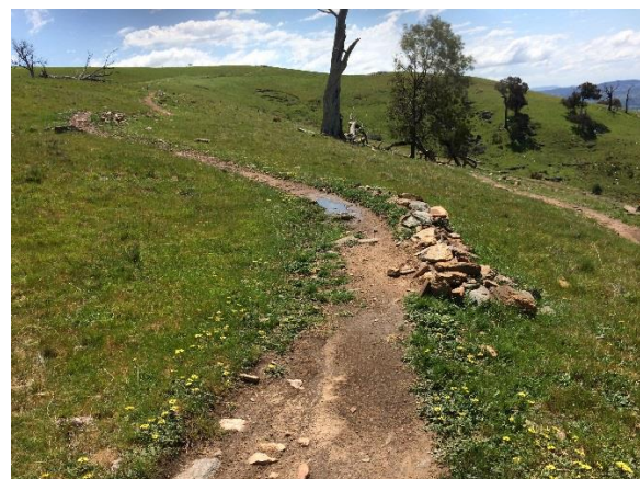
Image 2. These images show rocks used to line the existing trail. Any rocks that are not needed to prevent erosion should be relocated away from the trail
