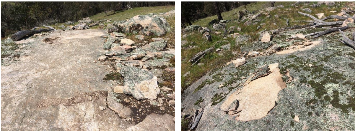
Image 3. (Left) Rock flakes (exfoliations) that have been broken and moved to create a smooth trail surface. (Right) rock flakes that have been destroyed leaving behind a visible scar. This damage looks more like vandalism than bike traffic.
