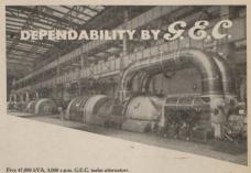
Five 47,000 kVA, 3,000 r.p.m. G.E.C. turbo-alternators in the Orlando Power Station of the Municipality of Johannesburg. A further live sets rated at 37,500 kVA are under construction for this Station. In the City Power Station of the same Municipality G.E.C. generating plant totalling 15,000 kVA is in
