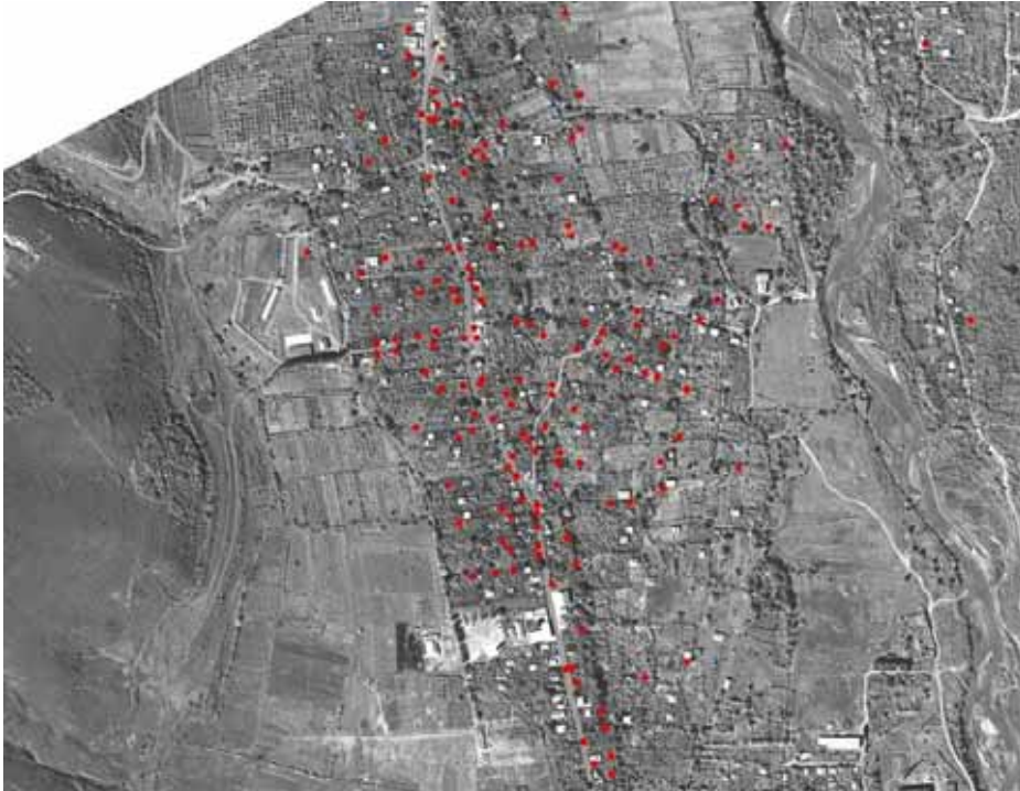
Satellite image of the Georgian village of Tamarasheni, South Ossetia, taken on 19 August. The red dots represent all buildings sustaining damage (152 structures in total). © 2008 ImageSat
