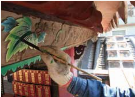
為簷板上色 Painting fascia boards
