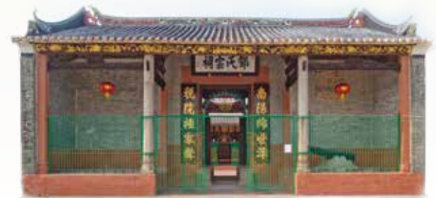
修復前、後的鄧氏宗祠 The Tang Ancestral Hall before and after restoration
