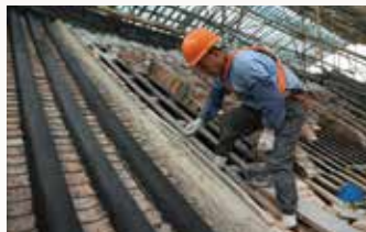
鋪砌天面瓦頂 Laying roof tiles
