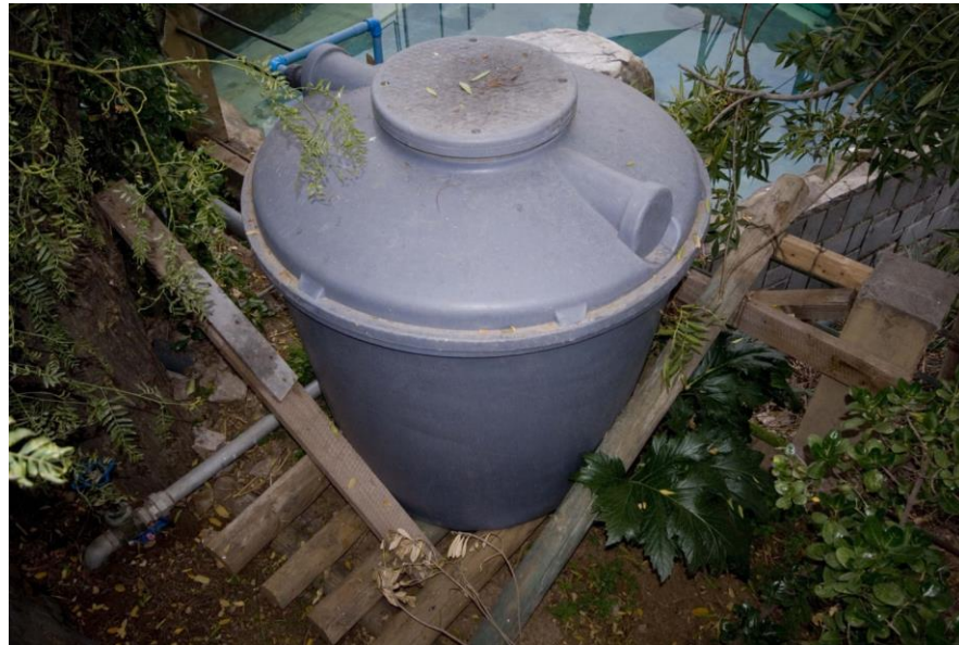
Figure 3. Water storage tank
