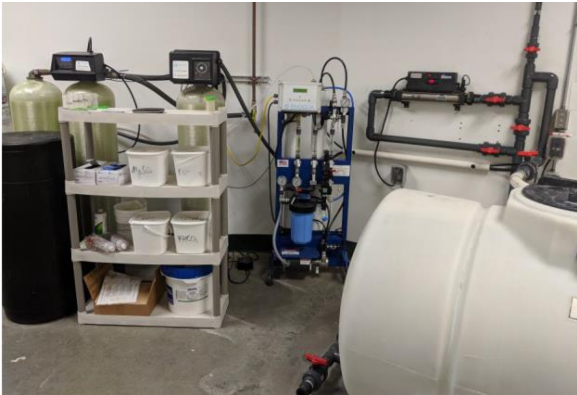
Figure 5: City source water is pre-filtered using a Reverse-Osmosis (RO) system ( along the wall ) and then reconstituted with appropriate salts and minerals ( visible on the shelf ) in the 300-gallon tank ( to the right ) for 30 minutes before distribution to holding tanks in each isolation room.
