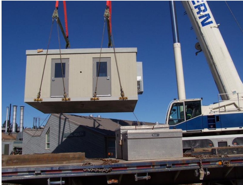
Figure 1. Moving the Amphibian Rescue Center onto the concrete pad
