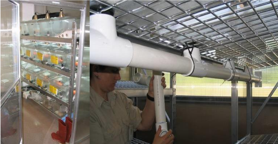
Figure 6. Left : Shelving with removable stand-pipe drains visible within the front of each polycarbonate enclosure. Right : The installation of the over-sized drain system under each shelf in the IAR; bulkhead from each enclosure fits within the “T” fitting below for passive flow when the interior standpipe is removed.
