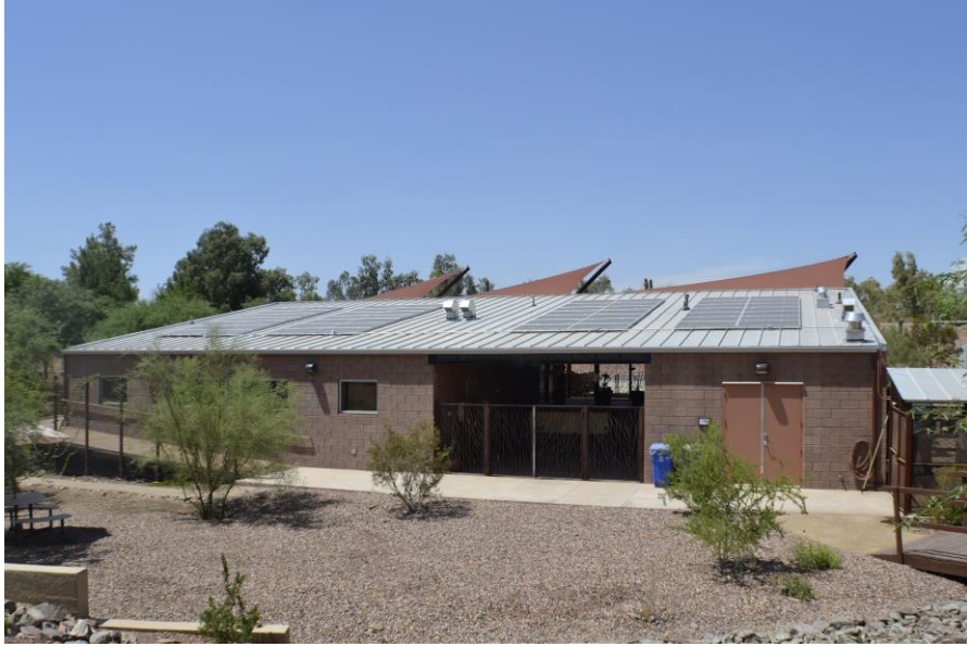
Figure 3. Exterior of the facility exhibiting solar panels
