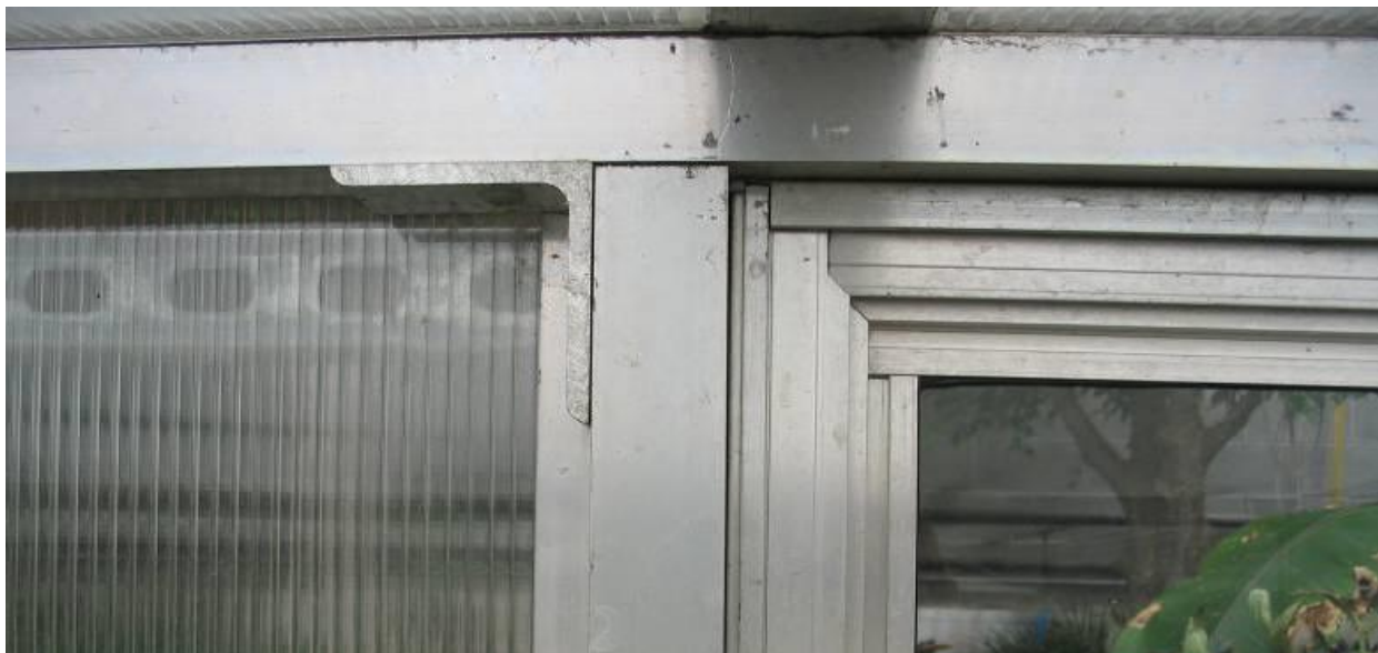
Figure 2. Close-up of the 1 in. (2 cm) aluminum angle pieces holding the 1.5x1.5 in. (3.8x3.8 cm) aluminum tubing and storm door.
