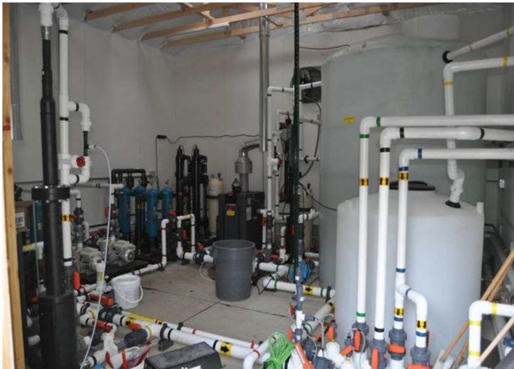
Figure 8. Interior view of stream life support system (LSS) building.
