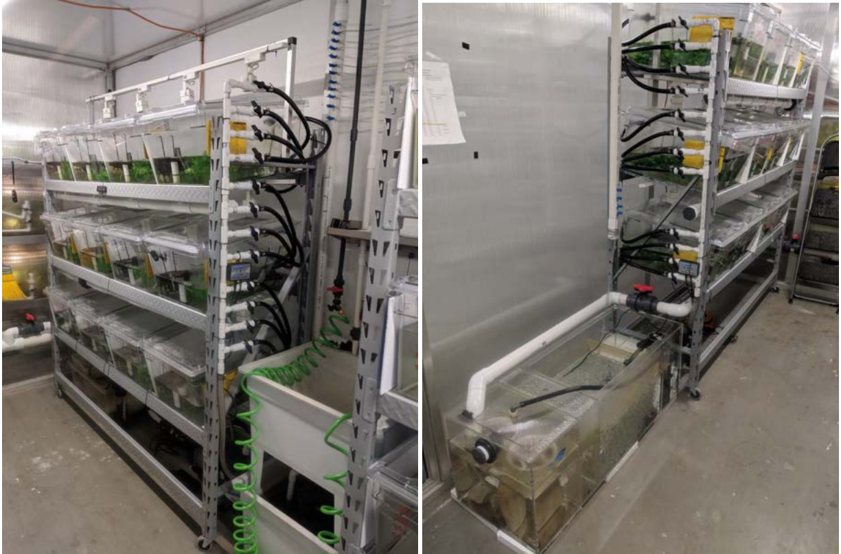
Figure 10: Specialized set-up for Mountain yellow-legged frogs ( Rana muscosa ) that provides improved water quality and allows water depths to vary 5-10" depending on breeding needs. Left: Flow through tubs with floating turtle docks for basking and feeding. Right: The sump houses filtration components such as K1 biological media, granular ferric oxide for phosphate removal, and filter socks as mechanical filtration.
