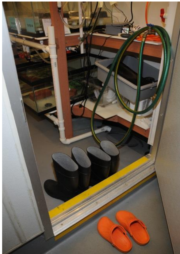
Figure 4. Elevated door threshold into an isolation room from common hallway. Note the dedicated footwear for hallway and each room.
