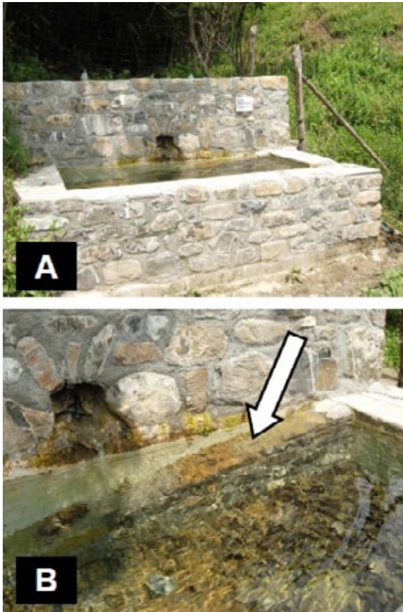
Figure 3. Purpose-built artificial sites for release of captive-bred individuals consist of stone washtubs (top) with a ramp to facilitate exit by metamorphs (bottom).
