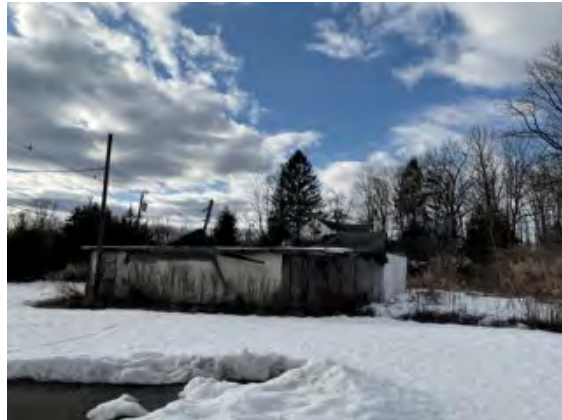
Lot 19 - Vacant Commercial Structure
