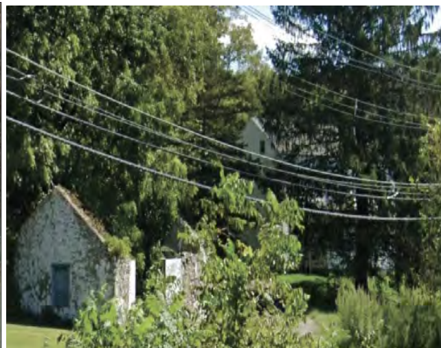
Lot 18 Residence, Shed/Residential Structure ( Source: Google)
