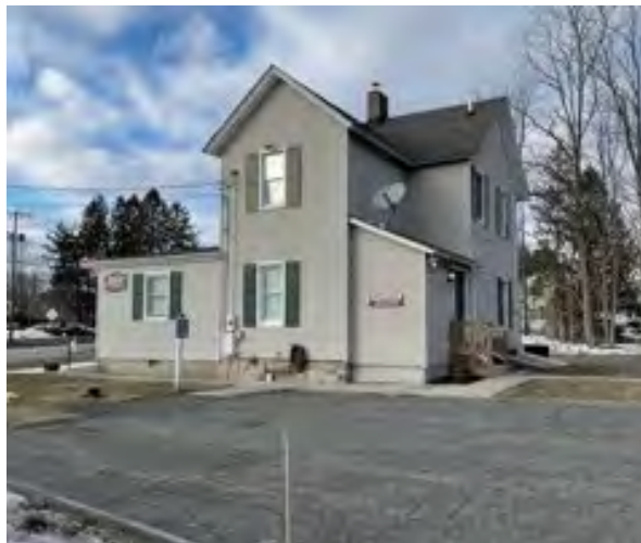
Lot 2 Commercial/Residential Structure
