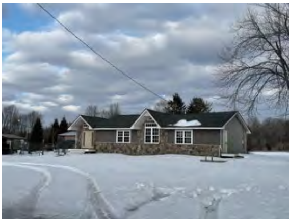
Lot 16 Commercial Office/Retail Structure
