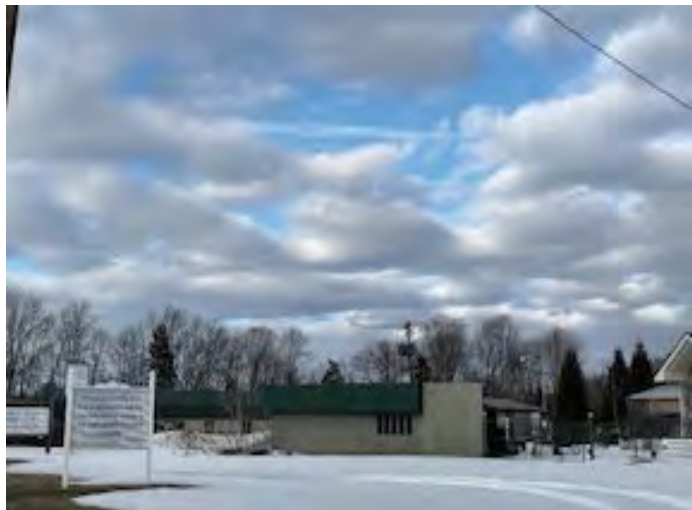
Lot 16 Commercial Storage Structure
