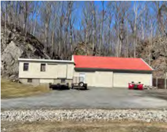
Lot 26: Public Garage Structure
