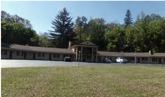
Lot 14.01: Motel Structure
