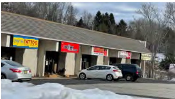
Lot 17.08: Commercial Strip Center
