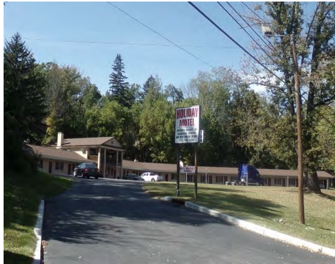
Lot 14.01: Motel Structure
