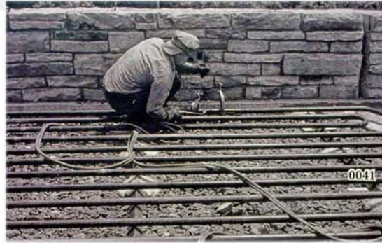
1/4" PIPE COILS 16" O.C.
