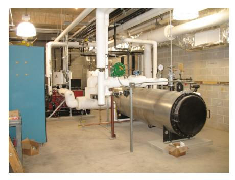
BioDiesel Engine Generator with Heat Recovery Equipment, MMCH C9
