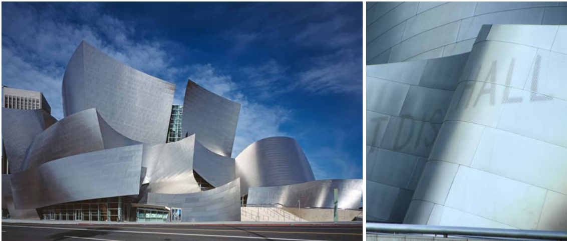
Figure 2-33 (Left) Disney Concert Hall by Frank Gehry (Right) Close view of the steel panels
