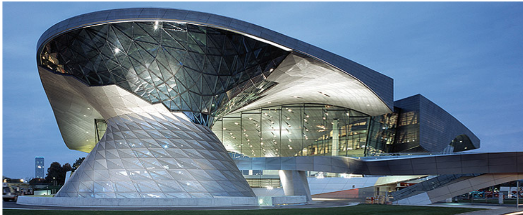
Figure 2-29 BMW Belt—a double cone surface, Munich, Germany 5
