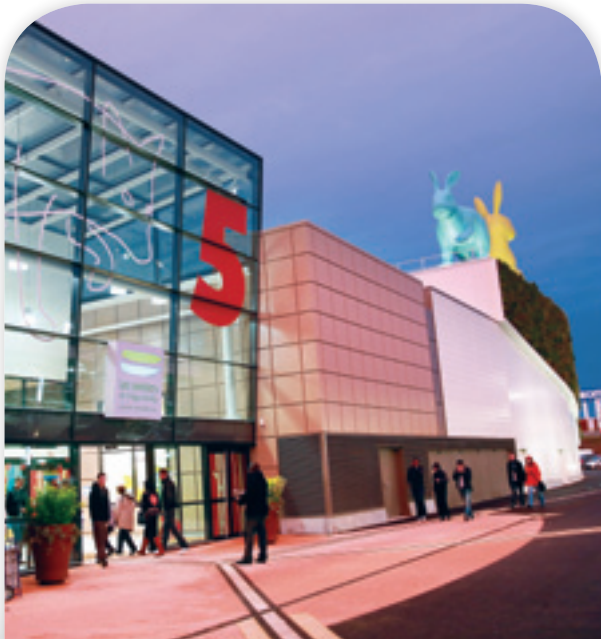
Les Sentiers de Claye-Souilly, entirely refurbished, already posted a 36% increase in footfall since its re-opening in November 2012.
