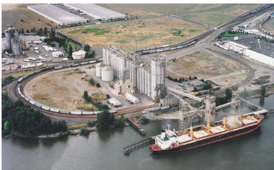
Facilities at Columbia Grain, Inc.
