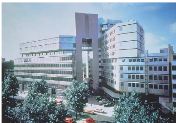
Commercial complex in Düsseldorf, Germany
