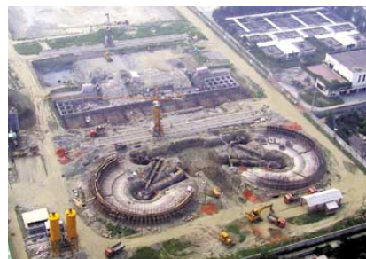
Construction of a water treatment plant in Chengdu, Sichuan Province, China
