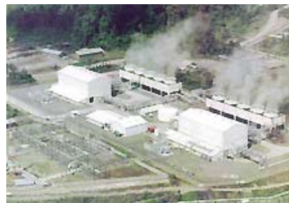
Mindanao Geothermal Power Plant in the Philippines
