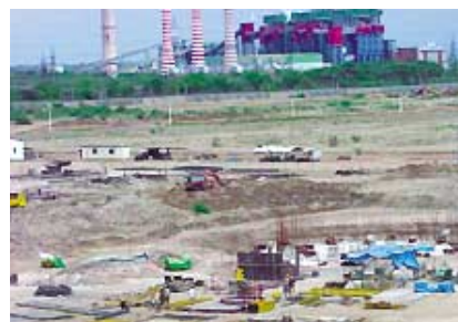
Coal-fired thermal power station project, under construction in Ramagundam, India
