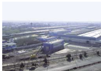
Passenger railway improvement project for Uzbekistan Railways
