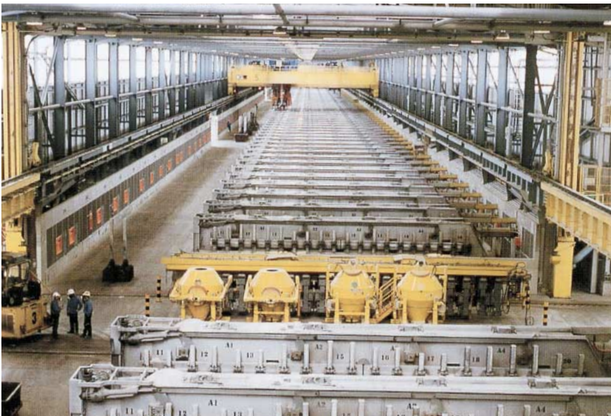
Boyne Smelters Ltd. Line 3 in Australia
