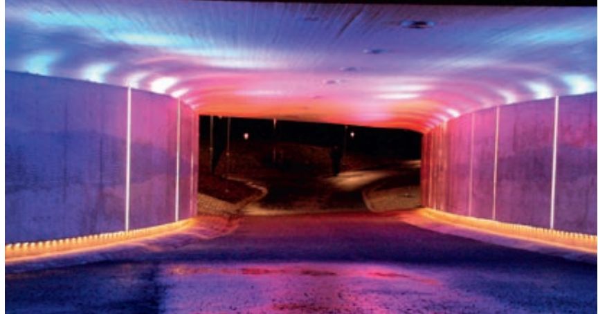
A collaboration project between business area Civil Engineering, the contractor, and business area Industry, which erected the lighting, has given the citizens of Linköping a unique lighting experience in the pedestrian and bicycle tunnel at the traffic roundabout Steninge. Using Fibonacci's sequences stage designer and light artist, Ulla Ridderberg, has contributed to the aesthetic experience. In daylight the combination of grey concrete and the lighting fixtures' glass rods creates a rather raw feeling but when night falls the glass rods light up in different color combinations and tempos depending on the time and season.
