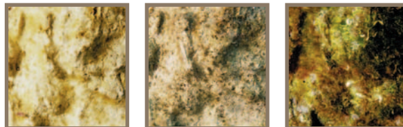
Right: the Digue Verte® (Grand Prize). Above: the roughness of the facing on the submerged part of the Digue Verte® fosters rapid colonisation by marine flora and fauna.
