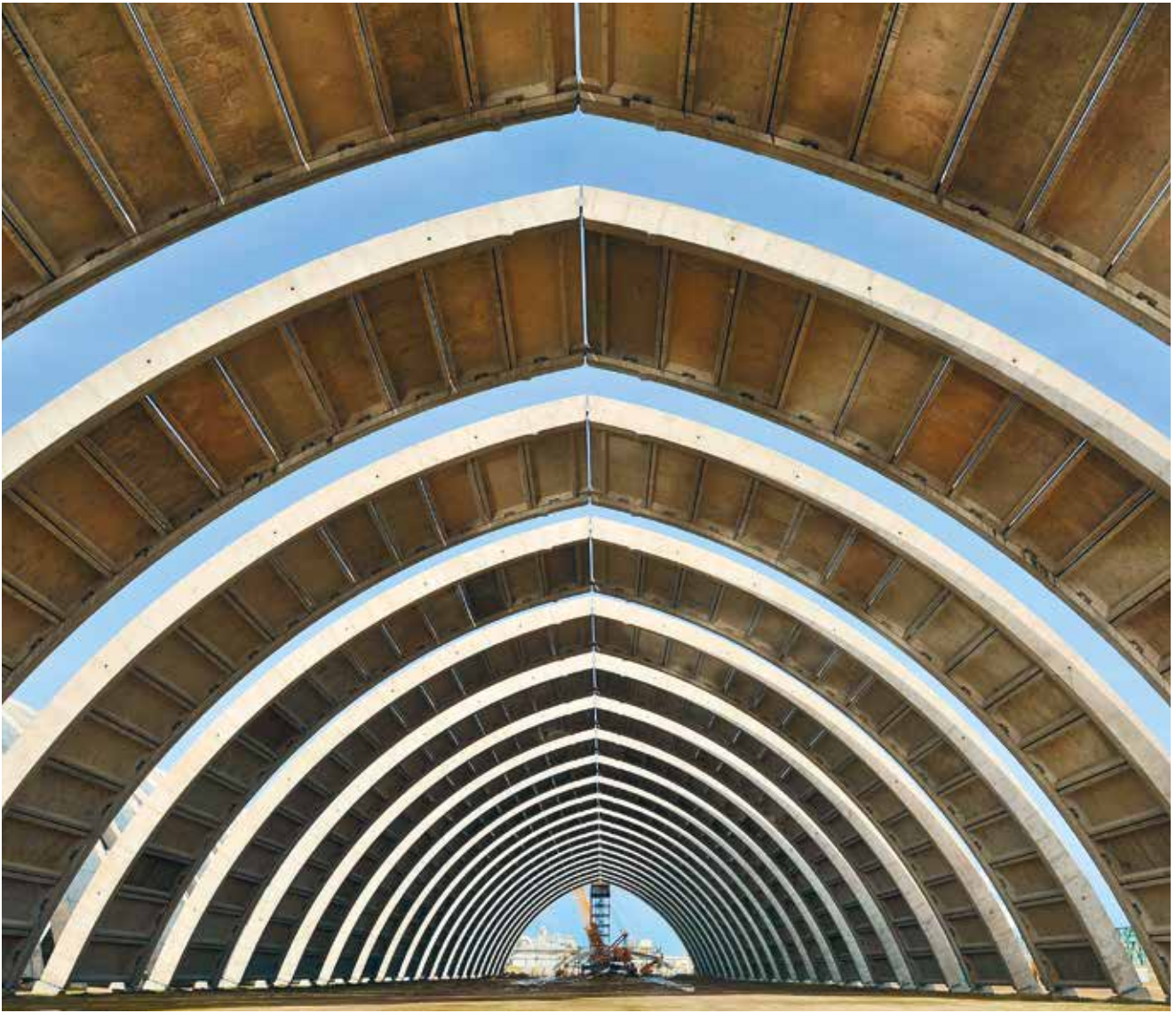
At OCP's Jorf Lasfar phosphate site in Morocco, Sogea Maroc built two phosphate fertiliser storage warehouses, each with a 100,000 tonne capacity.
