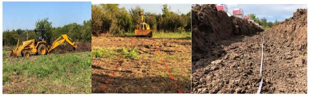
Figure 21. Trench excavation and preparation
