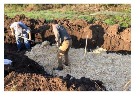
Figure 23. Researchers placing carbon in the trench
