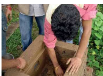
Figure 12. Making space by placing frames at 23 cm. from the bottom
