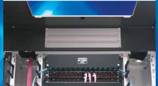
Internal view cooling corridor
