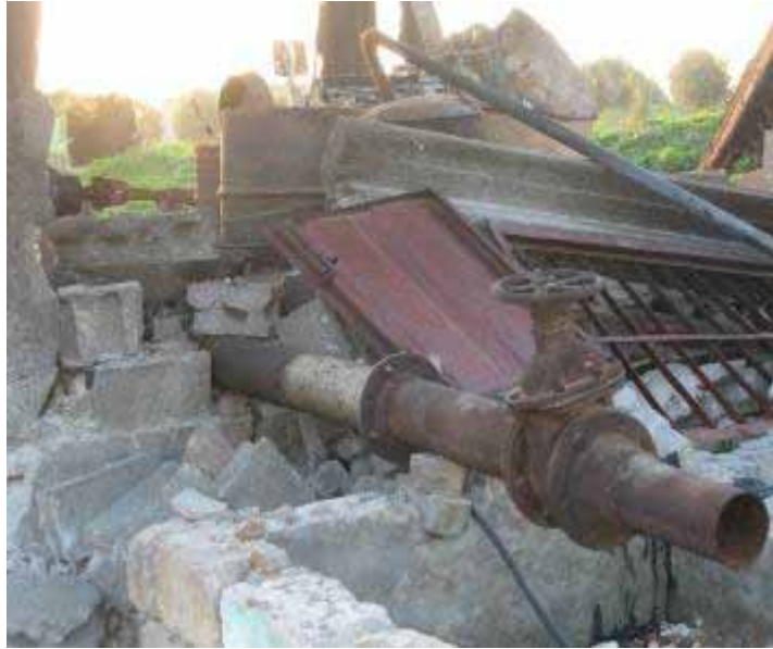
A water pump and well in the Zaytoun neighbourhood of Gaza City destroyed in an Israeli attack in January 2009 © AI
