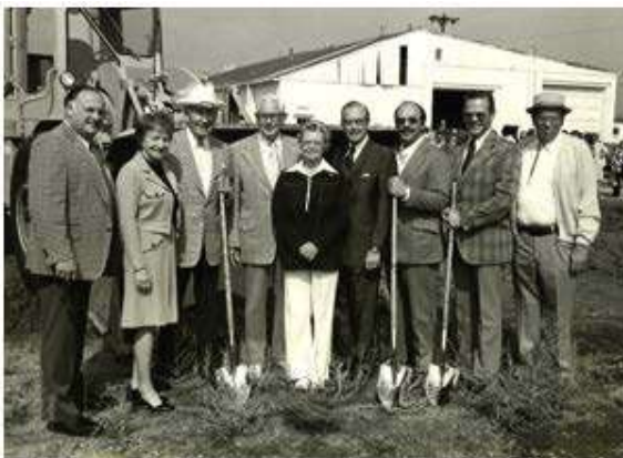
*Ground breaking of County Administration Building
