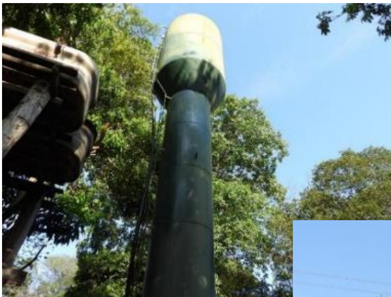
Figure 25 and 26. Water storage tanks for workers and also in surrounding communities.
