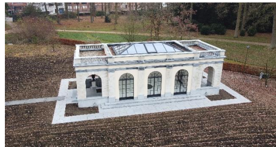
Photo 7. The Artois pavilion was completed in 2020.
