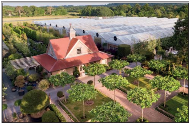
The Office. Leading to our Nursery
