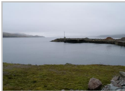
Pier at Furnace
