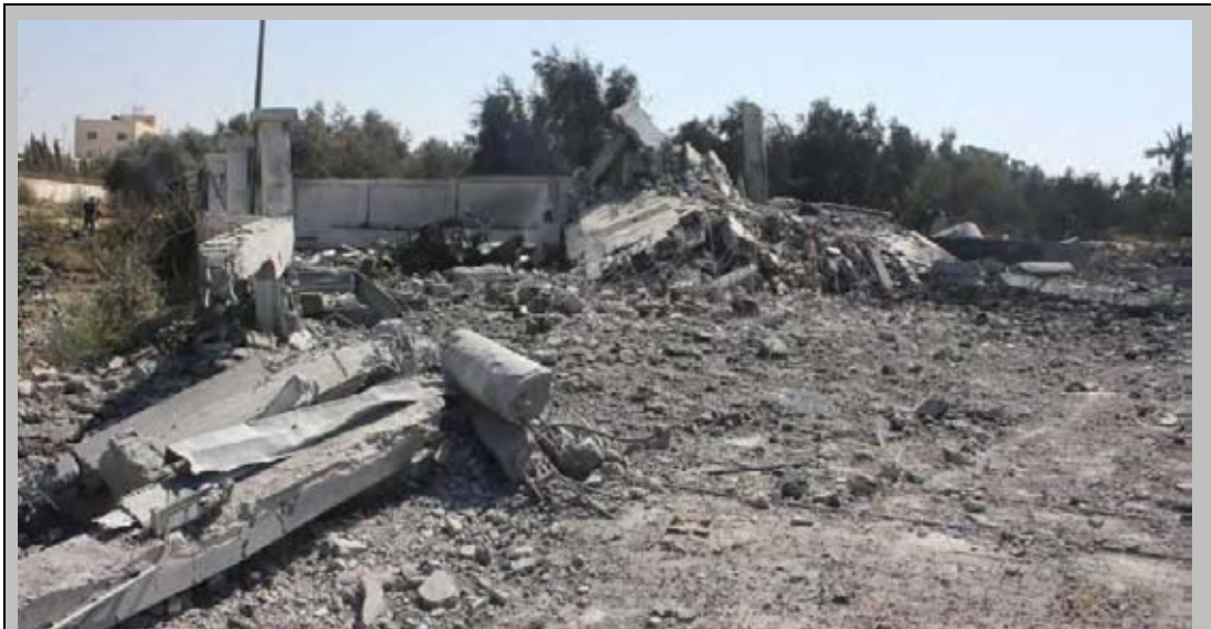
Photo 5.2.7: Al Nussirat sewage pumping station destroyed by Israeli jet-fighters
