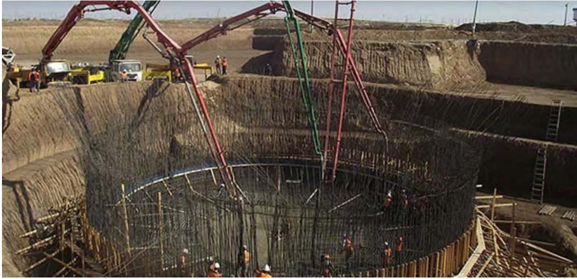
Photo 5.2.1: Implementing Phase, North Gaza Emergency Sewage Treatment (NGEST) Project
