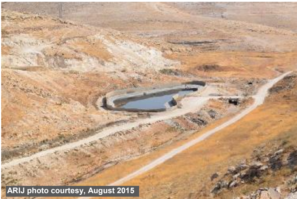
PHOTO 3.5: LEACHATE PRODUCED FROM SOLID WASTE - EL 'EIZARIYA LANDFILL
