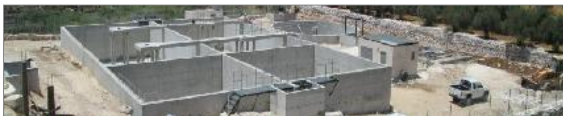
PHOTO 2.3: SAIR WASTEWATER TREATMENT PLANT DURING CONSTRUCTION PHASE
