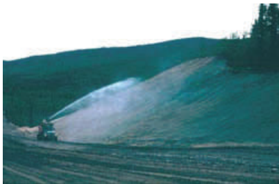
Figure 3 A typical cut slope being hydroseeded in Interior Alaska.
