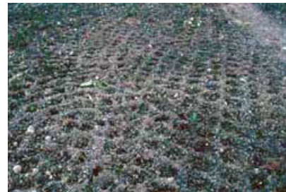
Figure 103: The imprinted pattern on the surface of the gravel pit. The pock marks trap moisture and seed. The steel wheels of the compactor (sheep’s foot) on the hard surface loosen the soil, forming a more vegetation-friendly condition.
