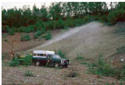
Figure 87: A small tow-behind hydroseeder in use.
