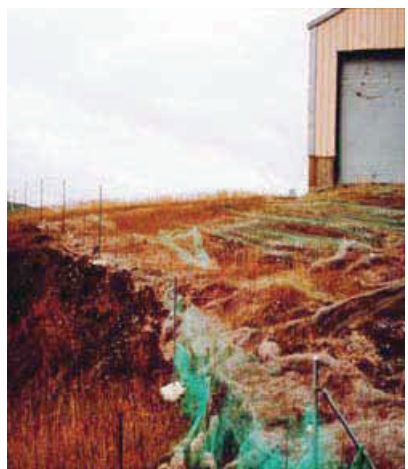
Figure 91: The plastic web or backing has created traps that have ensnared birds and fish - the use of this product should be carefully considered and based on true need and area of use, considering potential consequences.
