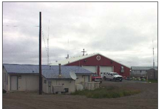
Atqasuk Fire Station
