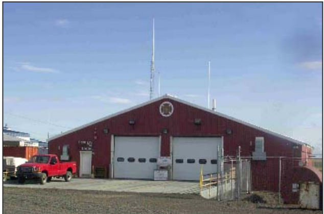
Point Lay Fire Station
