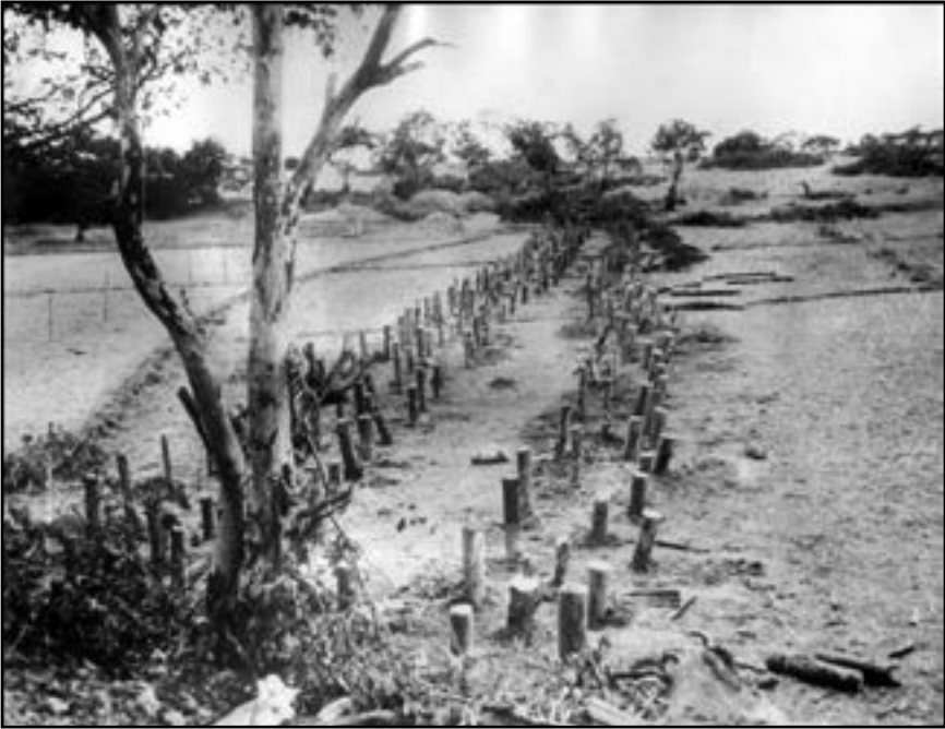
Figure 9.4. Improvised tank traps on Bataan akin to defensive measures taken by the PACR in Sector B. Courtesy of the National Archives and Records Administration.
