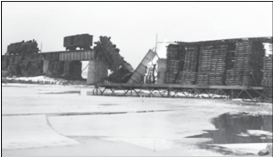
Figure 13.10. Hungnam destruction, 15 December 1950. Courtesy of the National Archives and Records Administration.
