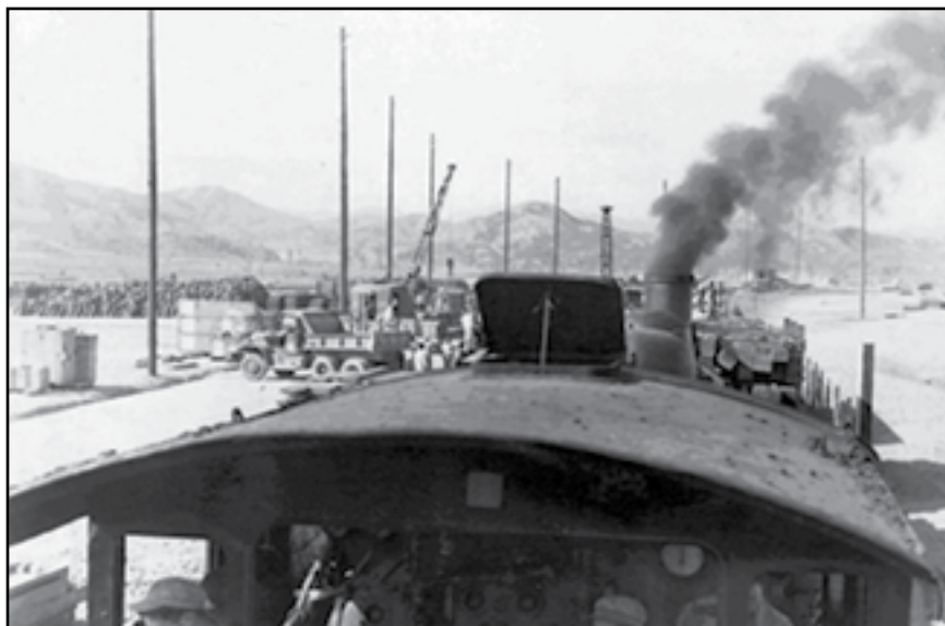
Figure 13.17. Supply train arrives at the 1st Marine Division Railhead at Wonju after reconstruction of the Killachon Bridge. Courtesy of the National Archives and Records Administration.
