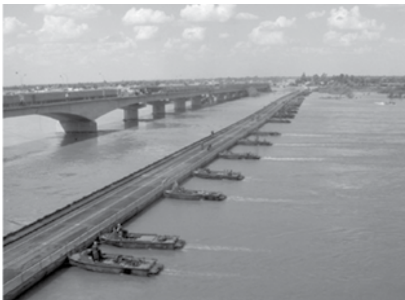
Figure 11.3. Birthday Bridge over the Tigris River. From Engineer , July–September 2003.
