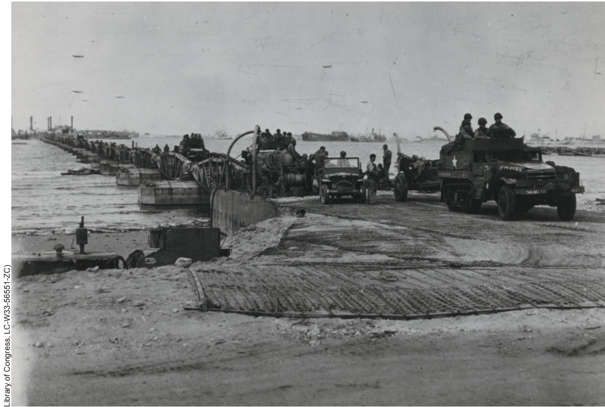
Mulberry harbor assembled in preparation for the invasion of Normandy, with military vehicles crossing a floating roadway, Cherbourg, France, 1944.
