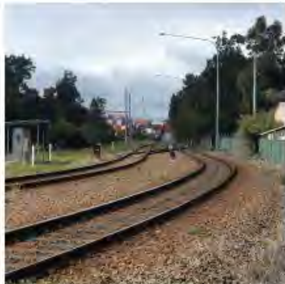
Above - Botany Yard, facing the Port connection
