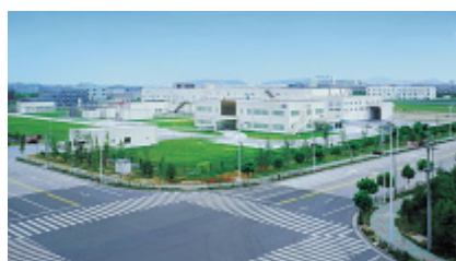
New APS™ assembly plant in China
