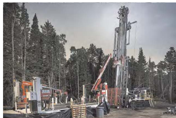
Drill Rig at Hidden Treasure project
