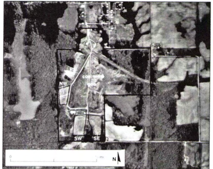
FIG. 8. 1982 aerial photograph of the Earthline landfill site.
