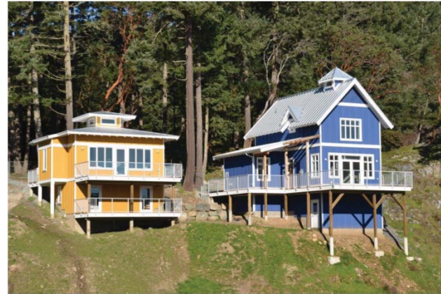
ASC Building Products – Spirit Bay, AK Project
