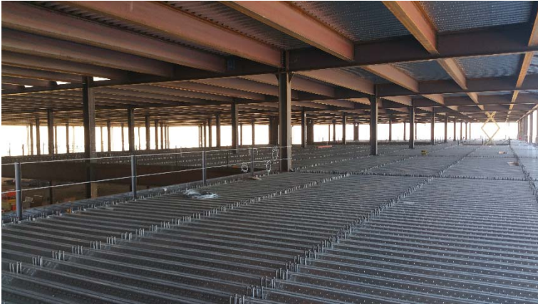
Tesla's Gigafactory -Sparks, Nevada
