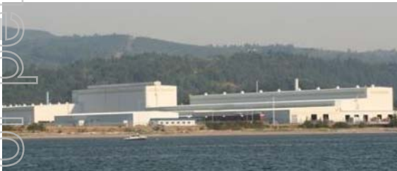
Metal coating & painting facility, Kalama, WA
