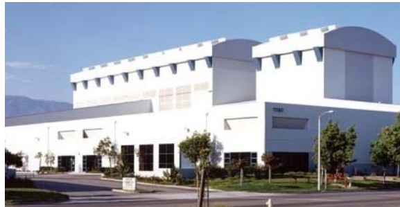
Metal coating & painting facility, Rancho Cucamonga, CA
