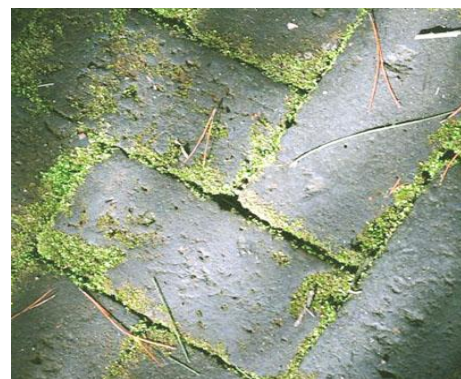
Fig. 3. Linear bryophytes in the joints of slabstone
