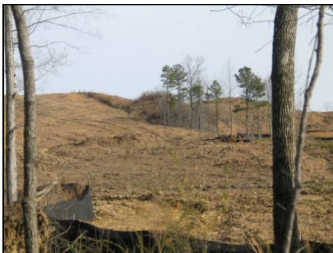
clearing land for development near Pell City
