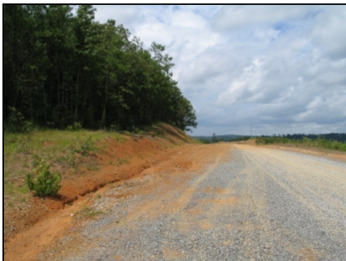
road construction for new development near Pell City
