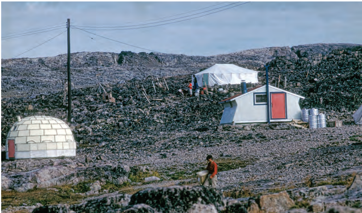
FIGURE 8.11 “Nunavut, 1960.” Most of the early forms of built heritage in the Arctic (some experimental) have been removed or repurposed to make way for more contemporary designs. Pictured here are three types of housing: a Styrofoam igloo, a prefabricated wooden house, and a canvas tent. Photograph by Rosemary Gilliat Eaton. Library and Archives Canada, Rosemary Gilliat Eaton fonds, Arctic travel series, e010835896 (item no. 4424960).
