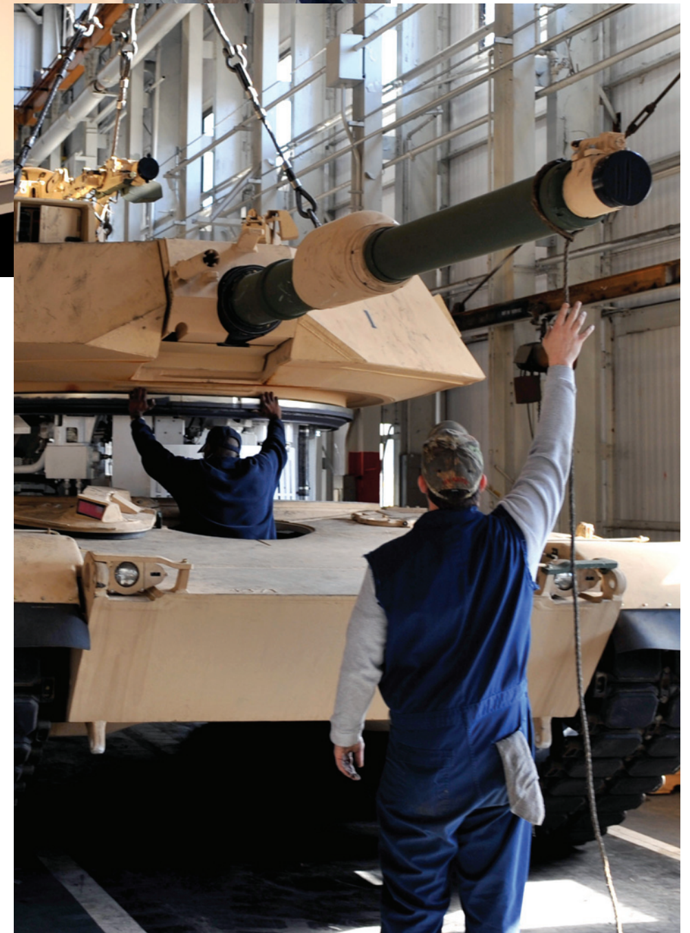
Mechanics at Anniston Army Depot marry a turret with its hull. Photo by Jeremy Guthrie
