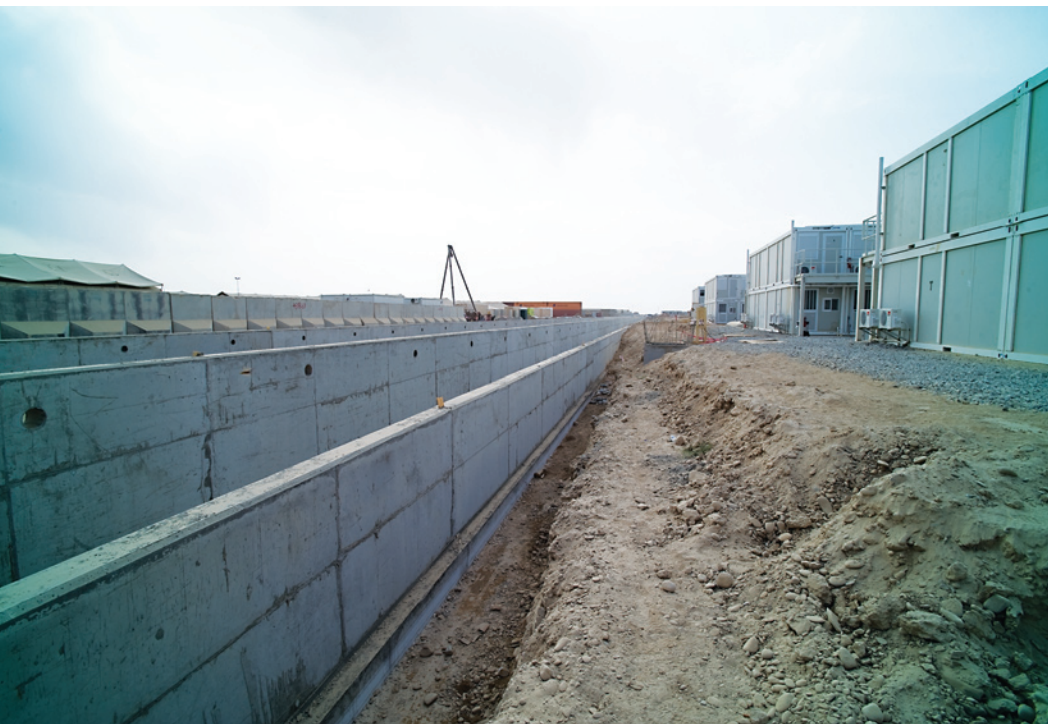
To expand living space, a concrete channel diverts the natural flow of a wadi that runs through NATO's Kandahar base.
