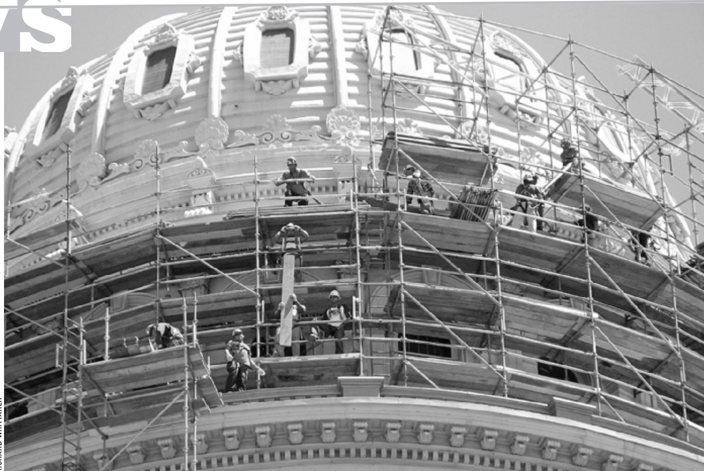
Prepping for paint: Workers set up scaffolding around the Capitol dome before adding a new coat of paint to spruce up the historic structure.
