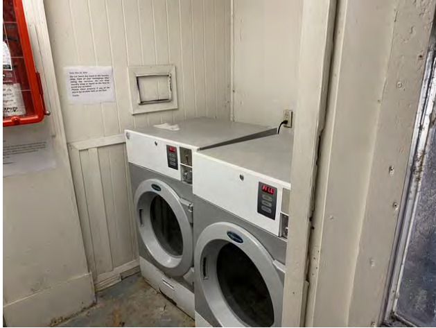
Central laundry facility
