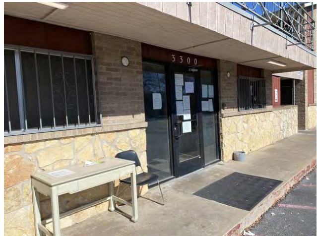
Leasing office exterior
