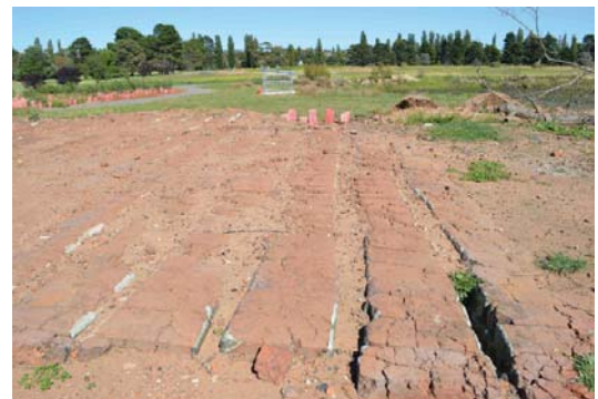
Floor of the kiln from the old brickworks with a new bird-hide under construction in the background.
