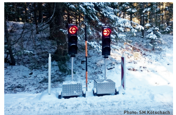
Entry point into the alternating one-way system, coming from Frohn. Two MPB 1400 signal heads show road users which direction can be used or when the road is blocked.
