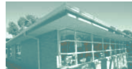
Upgraded facilities at The Australian Wine Research Institute
