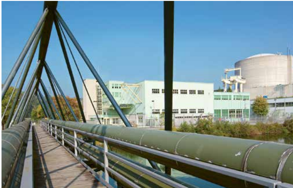
REFUNA pipe bridge over the Aare canal
