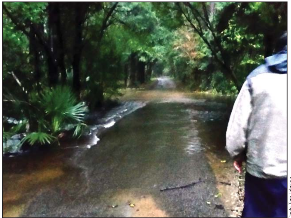
▼ Water flooding Tram Road and running through gardens.
